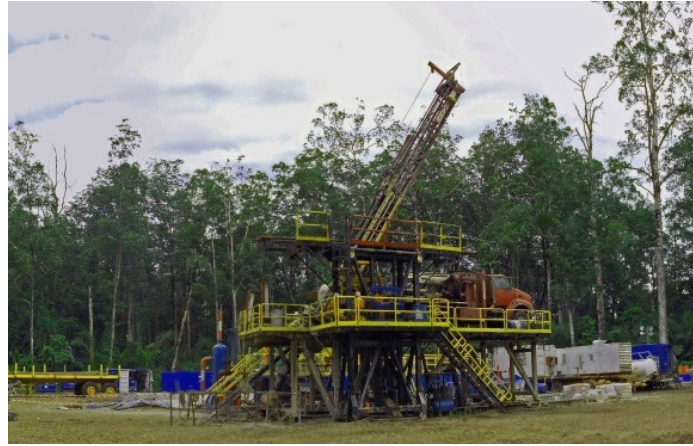
Schramm with sub-structure (tiled, USRD from slant well)
